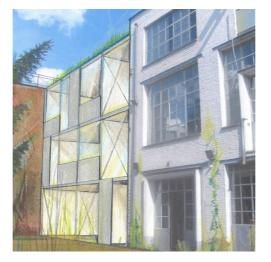
project: the ruinous existing barn is to be replaced by a tree storey high steel structure. as a reference to the original industrial usage of the building, structural façades are composed of large glass panels and prefabricated sandwich panels. the new vertical garden in the narrow backyard allows natural daylight to enter the rooms from a green oasis in this enclosed city area.
